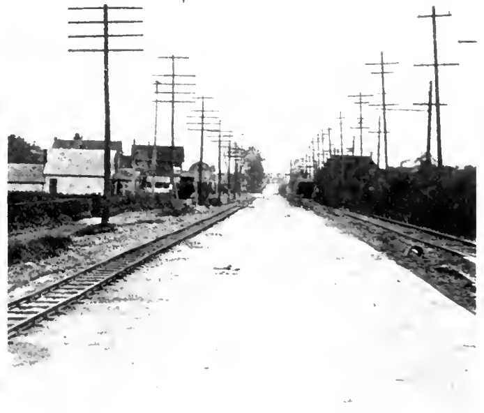
Fig. 2—The same section of road after the highway commission had done its work.
